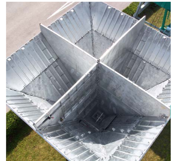
Storage bins, intermediate walls and discharge mouths fully heat galvanised
